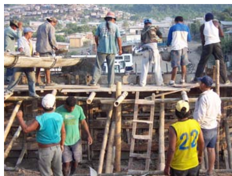
Workmen building the platforms
