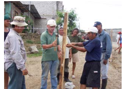
The fence being erected for the Church land.
